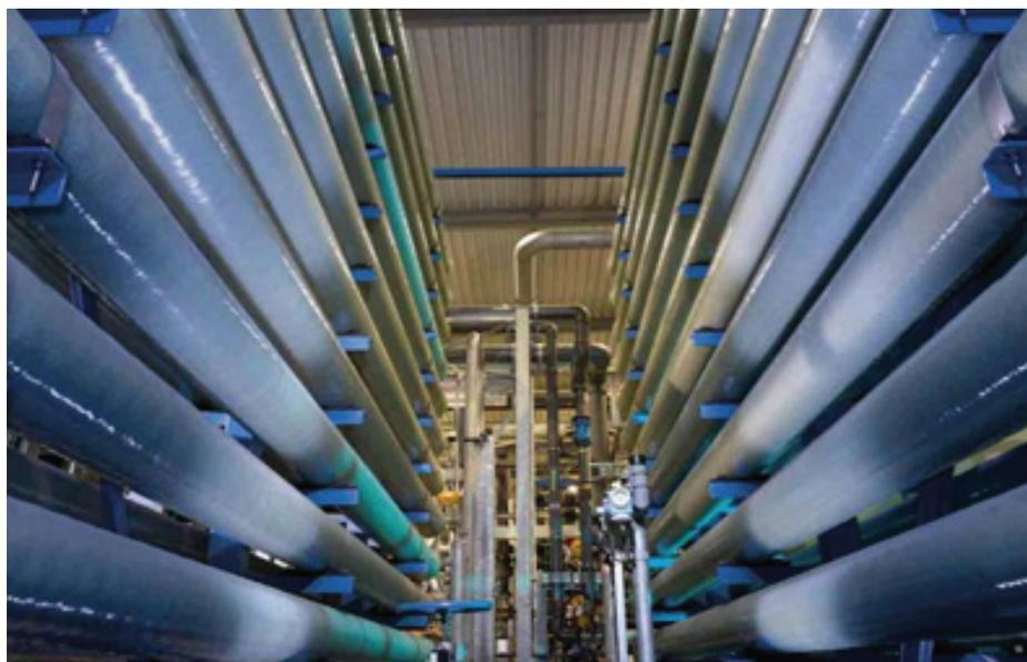
Pressure vessels housing reverse osmosis elements at DECO water treatment facility. (Photo courtesy of Evides Industriewater B.V.)
