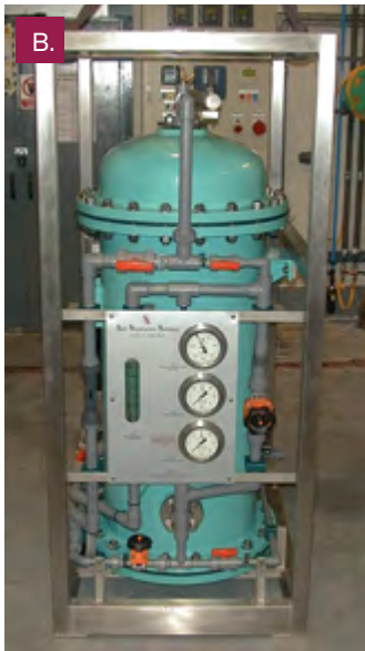
Figure 1. Images of Rothera plant (A. Sand filter and B. RO unit), courtesy of Salt Separation Services, UK.
