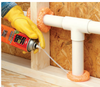
Seal pipe penetrations
