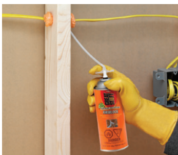
Seal Electrical Through Wall Studs
