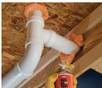
Seal pipe penetrations
