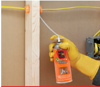
Seal Electrical Through Wall Studs
