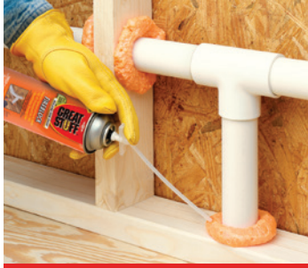
Seal pipe penetrations
