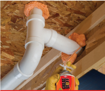
Seal pipe penetrations
