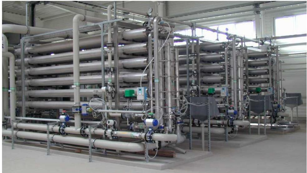
*VA Tech built a new water treatment plant using intermittent biocide dosage and fouling resistant membranes, rather than chlorine, to produce process water from a nearby river, the Weisse Elster. (Photo courtesy of Infra-Zeitz)*
