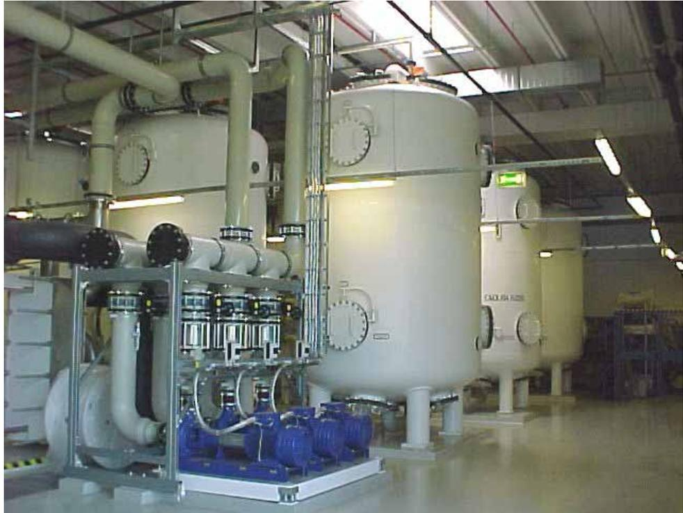
*The Fab 30 plant in Dresden, Germany, uses the UPCORE™ system in its demineralizer unit to reduce ions, silica, boron, and TOC levels in process water. (Photo courtesy of AMD)*
