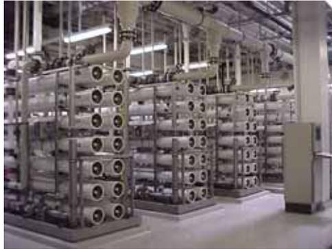
The RO unit uses FILMTEC™ SG30LE-430 semiconductor grade elements.
