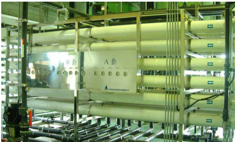
The increased surface area and element efficiency of FILMTEC™ BW30LE-440 elements increases flow rate, reduces fouling and prolongs service life. (Photo courtesy of OPTO Tech Corporation)
