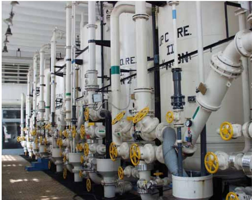
*The new UPCORE™ water-treatment system at the AES Tiszapalkonyai Hőerőmű power plant has been operating reliably since 1995. The system uses DOWEX™ UPCORE Mono ion exchange resins. (Photo courtesy of AES Tiszapalkonyai Hőerőmű)*
