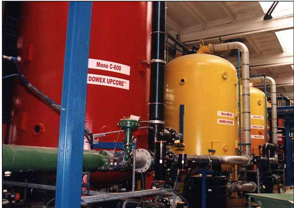
*At Polski Koncern Naftowy there are seven treatment lines for boiler feed water, all of which use the UPCORE™ system and DOWEX™ UPCORE Mono ion exchange resins. The photo above shows one of the lines with the cation bed in the foreground, then the weak base anion bed, and then the anionic layered bed. (Photo courtesy of Polski Koncern Naftowy Orlen)*
