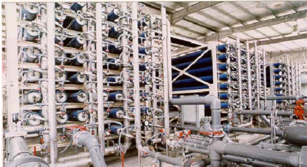
*SUT Seraya operates the reverse osmosis system that uses FILMTEC™ fouling resistant membranes to supply high quality industrial water to Singapore industry. This view shows the pressure vessel racks of three of the six reverse osmosis trains. (Photo courtesy of SUT Seraya.)*
