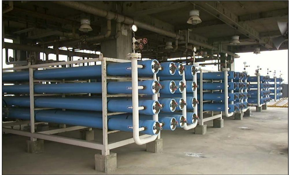
*The use of FILMTEC™ membranes enabled China American Petrochemical Co., Ltd. to reclaim wastewater, resolving water shortage problems during droughts. (Photo courtesy of CAPCO)*
