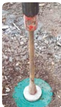
Picture 4: Sliding hammer inserted into.
